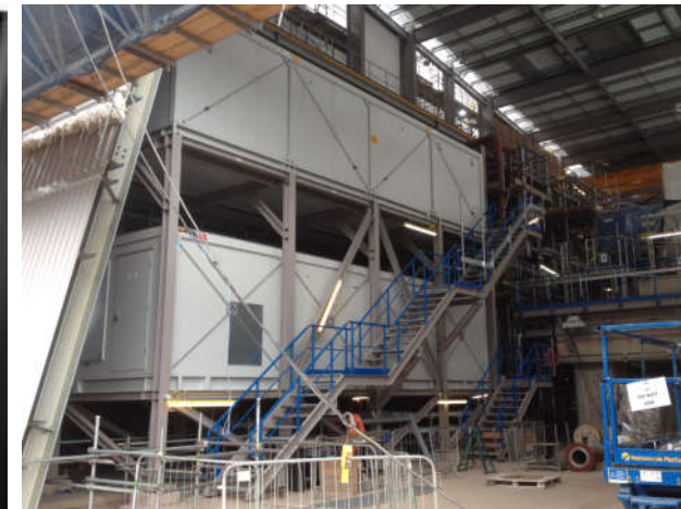
Two levels of E-Houses with stairs, platforms and handrails
