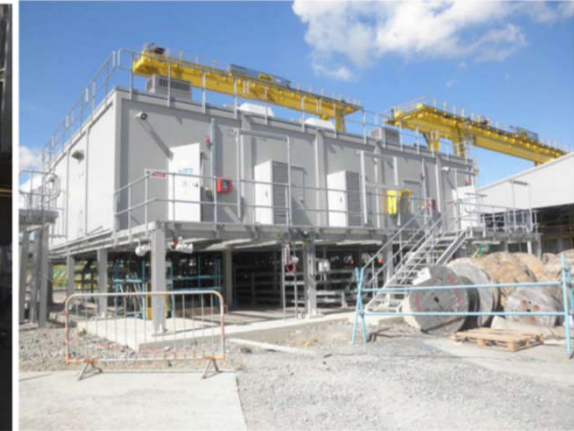
Steel support structure with stairs, platforms and handrails
